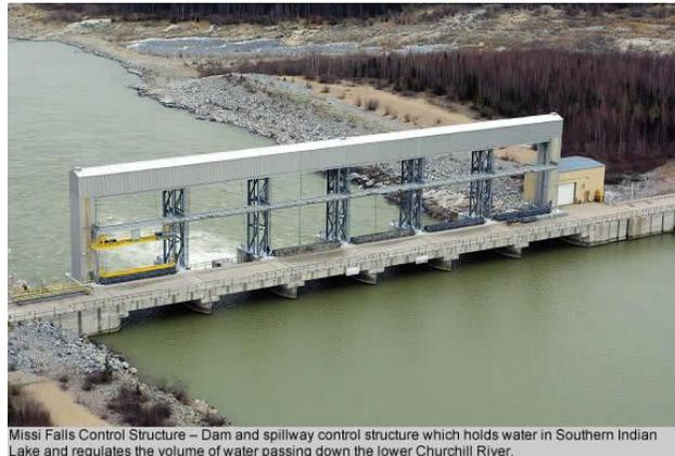
Missi Falls Control Structure – Dam and spillway control structure which holds water in Southern Indian Lake and regulates the volume of water passing down the lower Churchill River.
